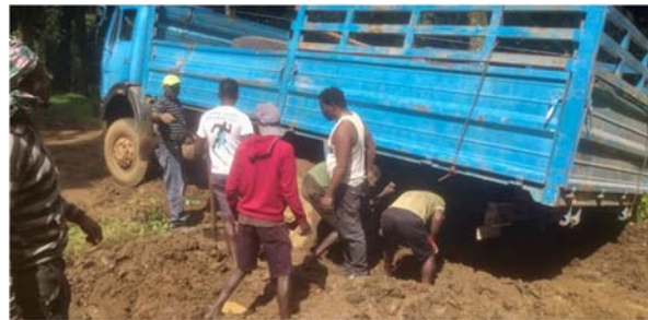
The Maji District officials arranged for other road repair as well, but heavy rains were sometimes too much on a road that was graded, but not graveled.
